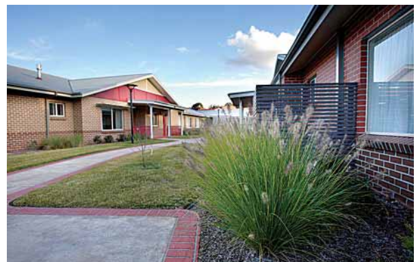
Hammond Care specialises in aged and dementia care. Their new 'Southwood' at Hammondville is a six cottage nursing home purpose-built for people with dementia. The domestic design aims to support the residual skills of residents.
